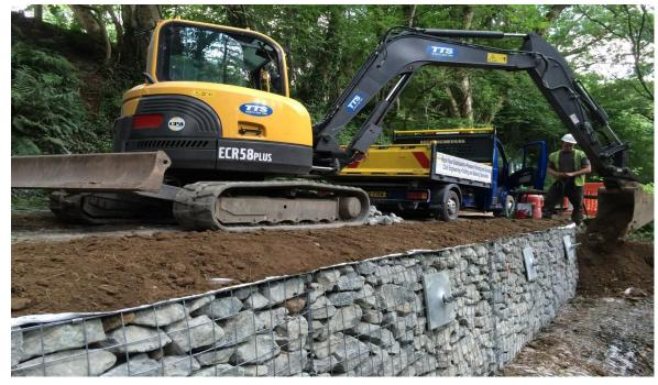
The works consisted of the stabilisation of a sheer slope which supports and existing highway. Soil nails were used to stabilise the slope and gabion baskets installation to support the existing highway.
